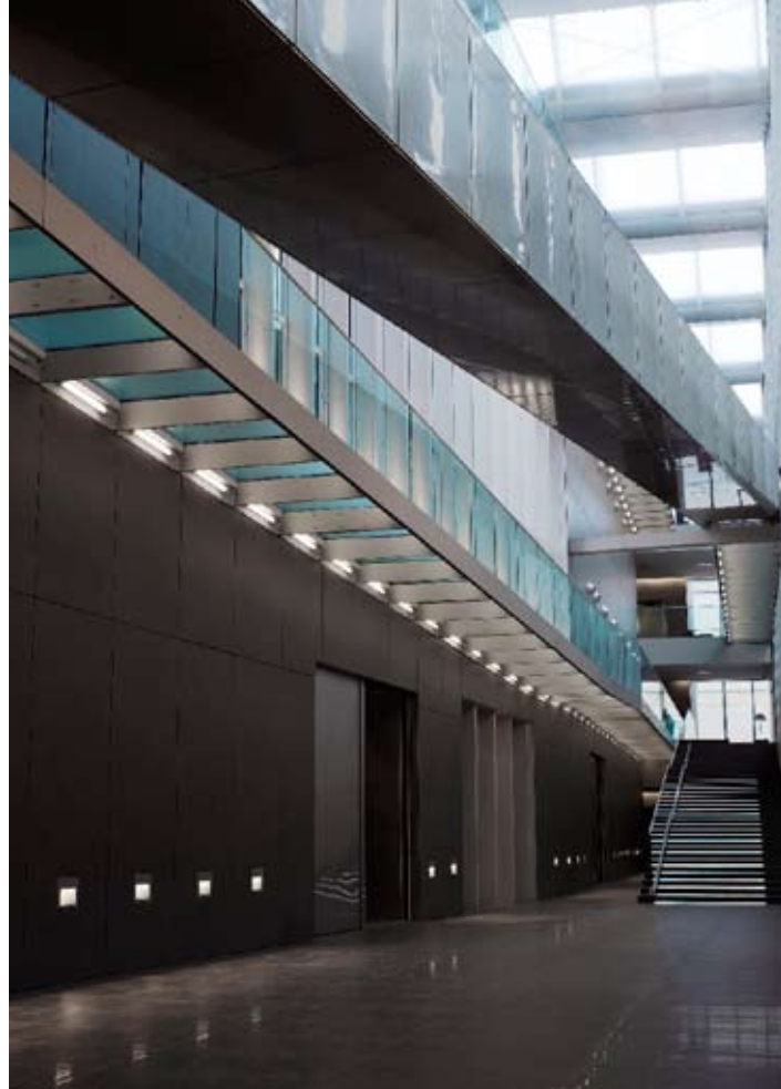
Suspended glass walkways and bridges with steel girders link the various spaces that are distributed over four levels and generously illuminated by the large skylights. On the previous page, "Wollen" by Michelangelo Pistoletto hangs at the entrance of the building and links the brand to its roots in Biella
